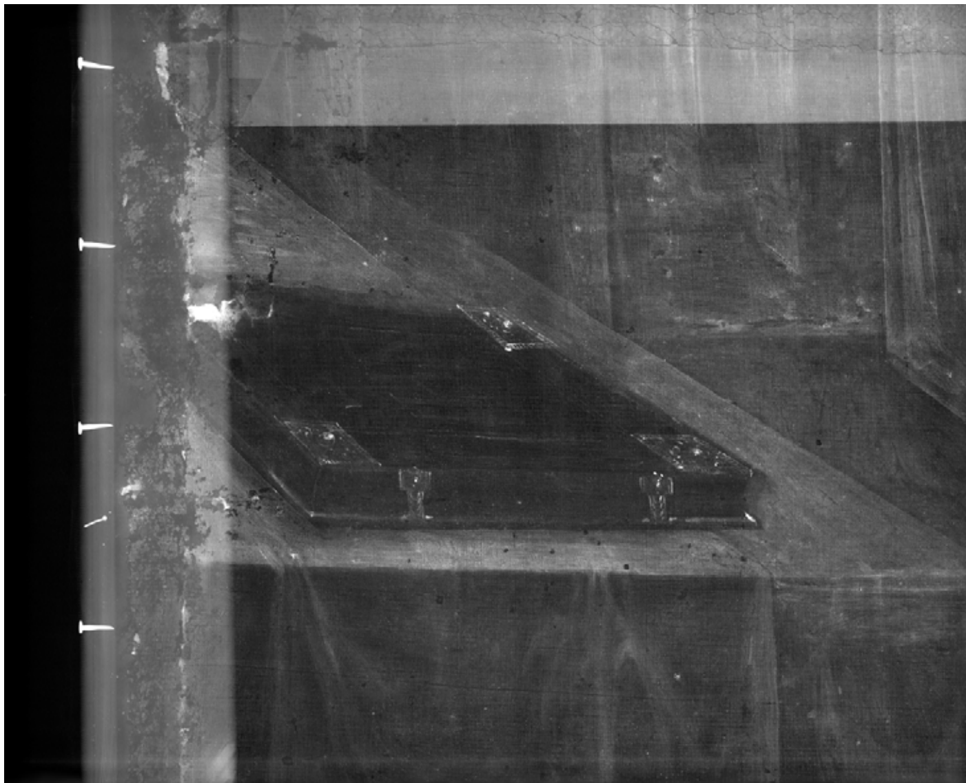
Detail v RTG
